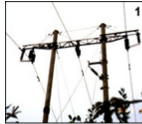
(35kv MOA without gaps for middle phase)
