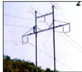
(110kv MOA with gap for dead-end tower)
